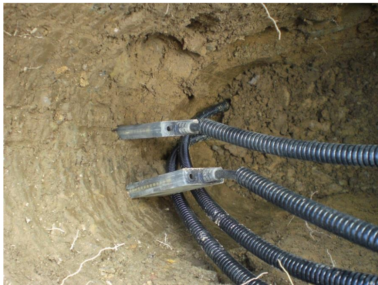
Figure 11: Inserted sensors and backfilling
