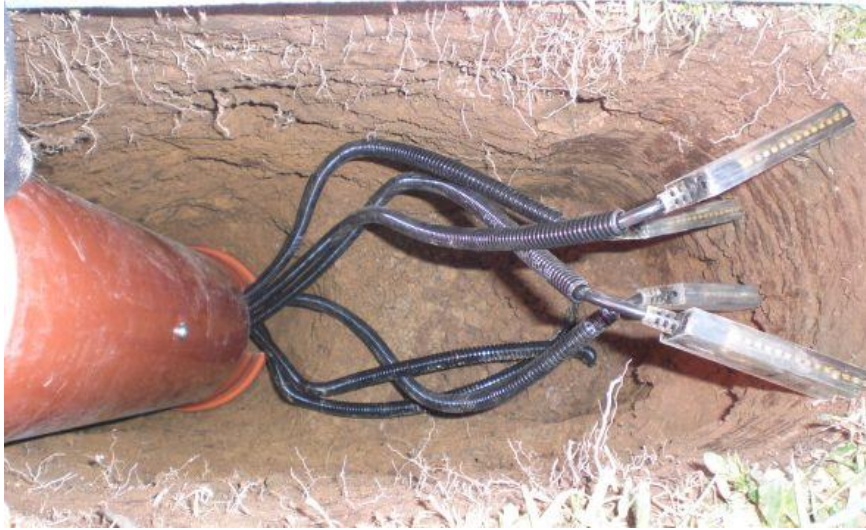
Figure 14: Cable guiding
