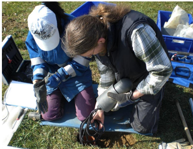
Figure 17: "Screwing" the End-Device into the KG-pipe
