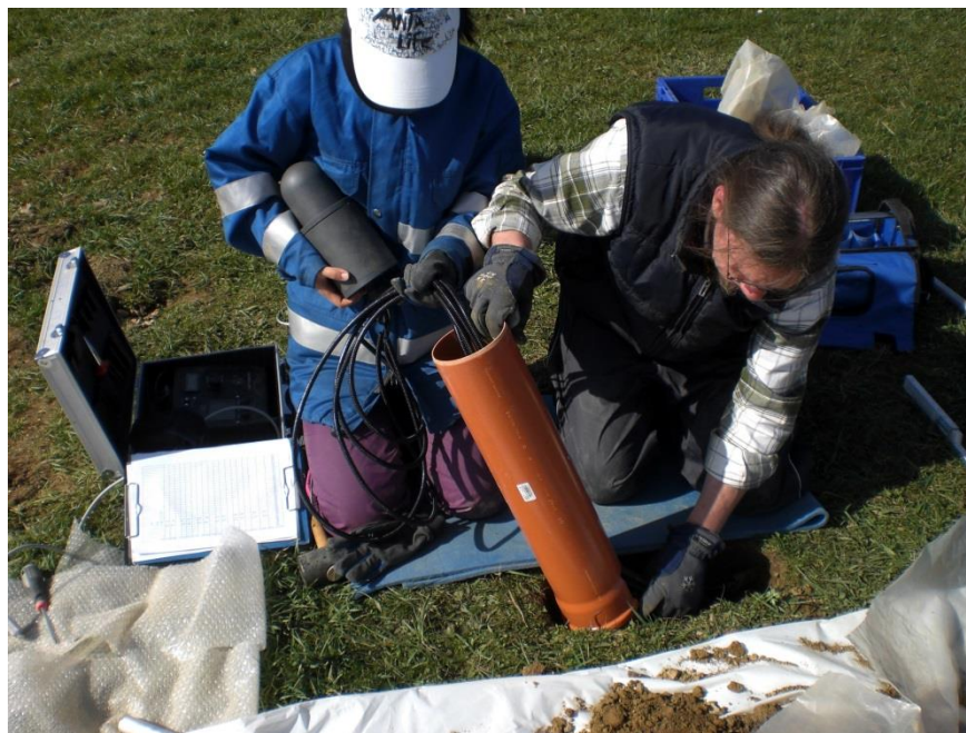
Figure 13: Inserting the KG pipe
